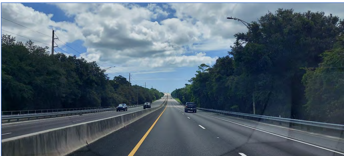
S.R. 116 (Wonderwood Expressway)
