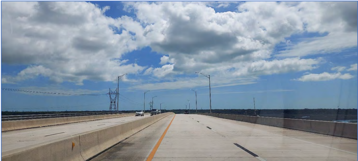
S.R. 116 (Wonderwood Expressway)
