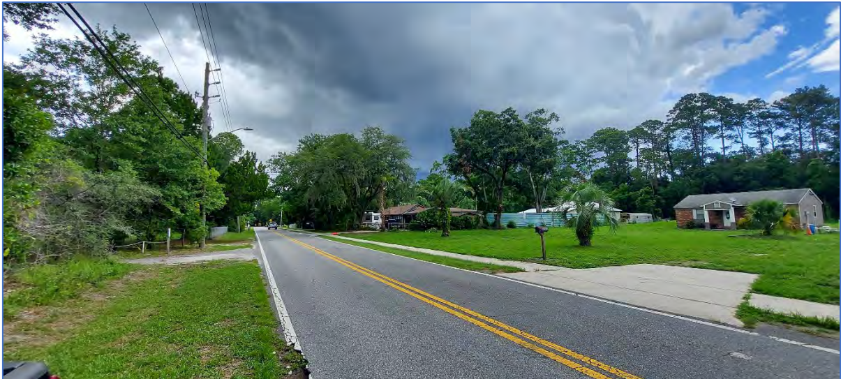
Bowden Road, north of Belfort Road
