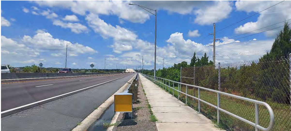
S.R. 116 (Wonderwood Expressway)
