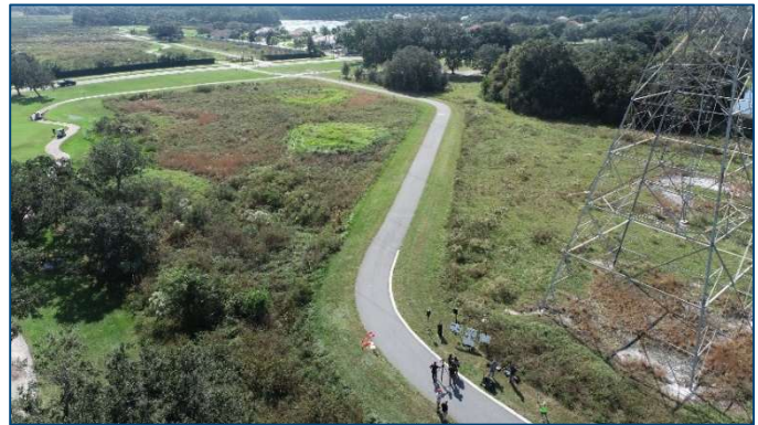
An aerial view of the Starkey Park Trail, which connects to the Suncoast Trail. Note the high power transmission tower on the right. Source: Florida Greenways and Trails Foundation
