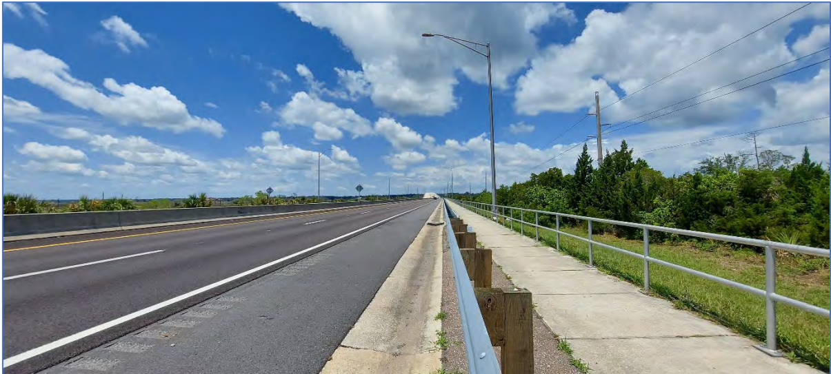
S.R. 116 (Wonderwood Expressway)
