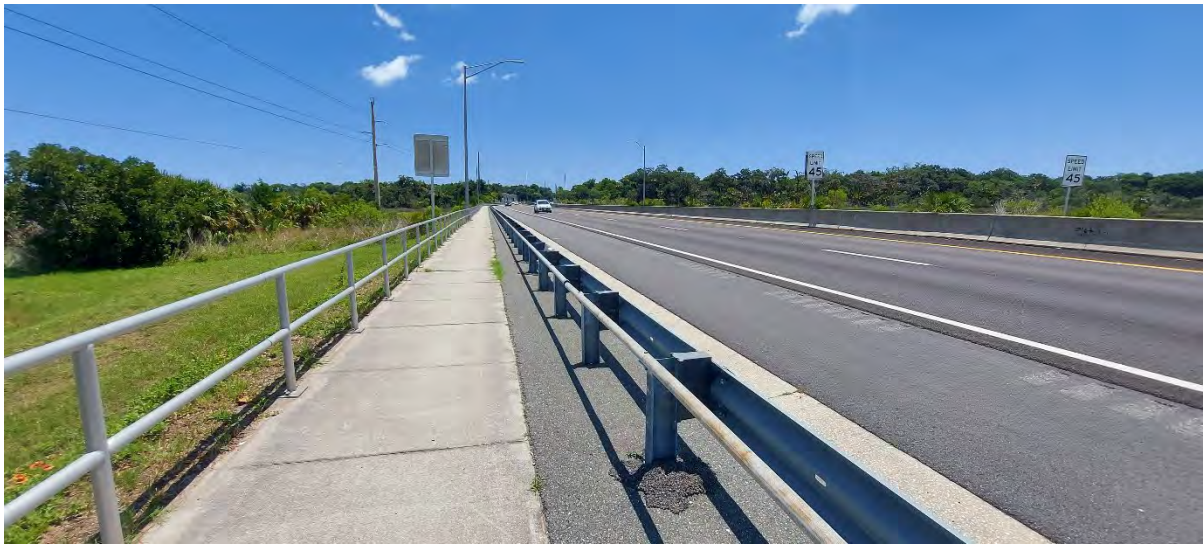
S.R. 116 (Wonderwood Expressway)
