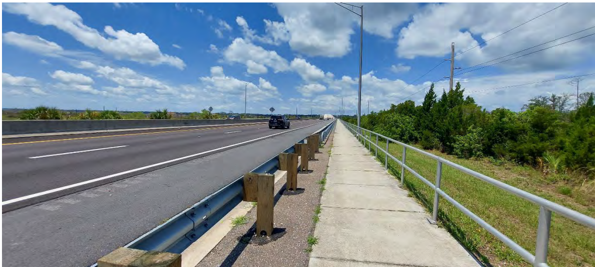
S.R. 116 (Wonderwood Expressway)
