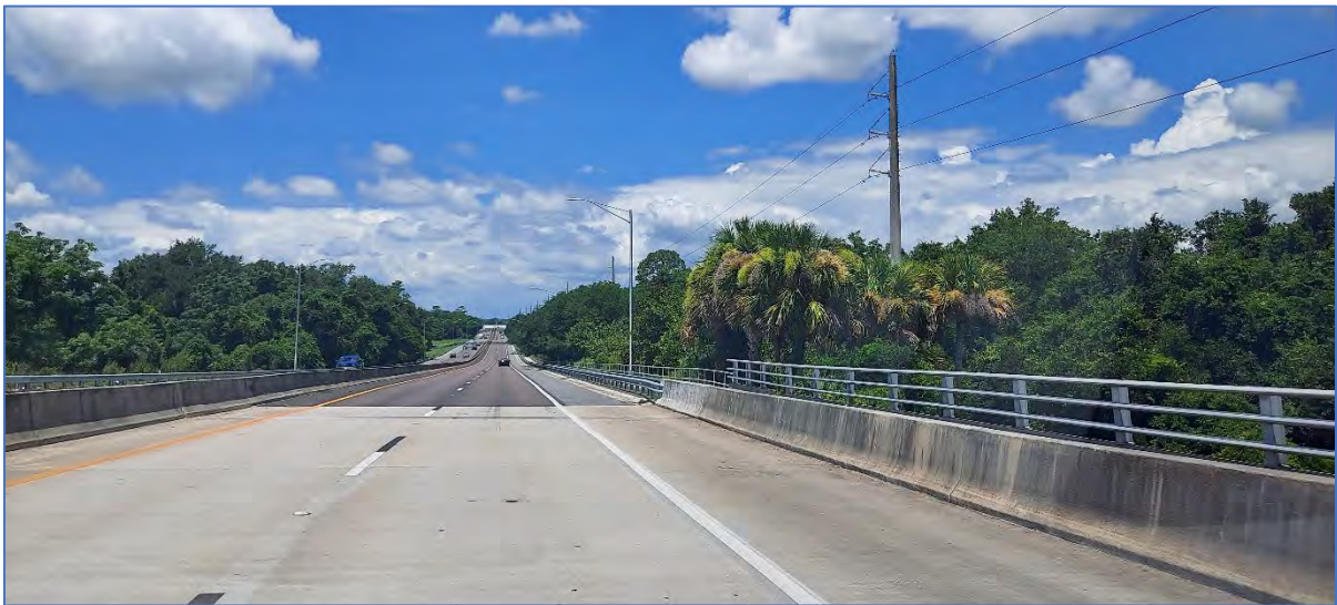
S.R. 116 (Wonderwood Expressway)
