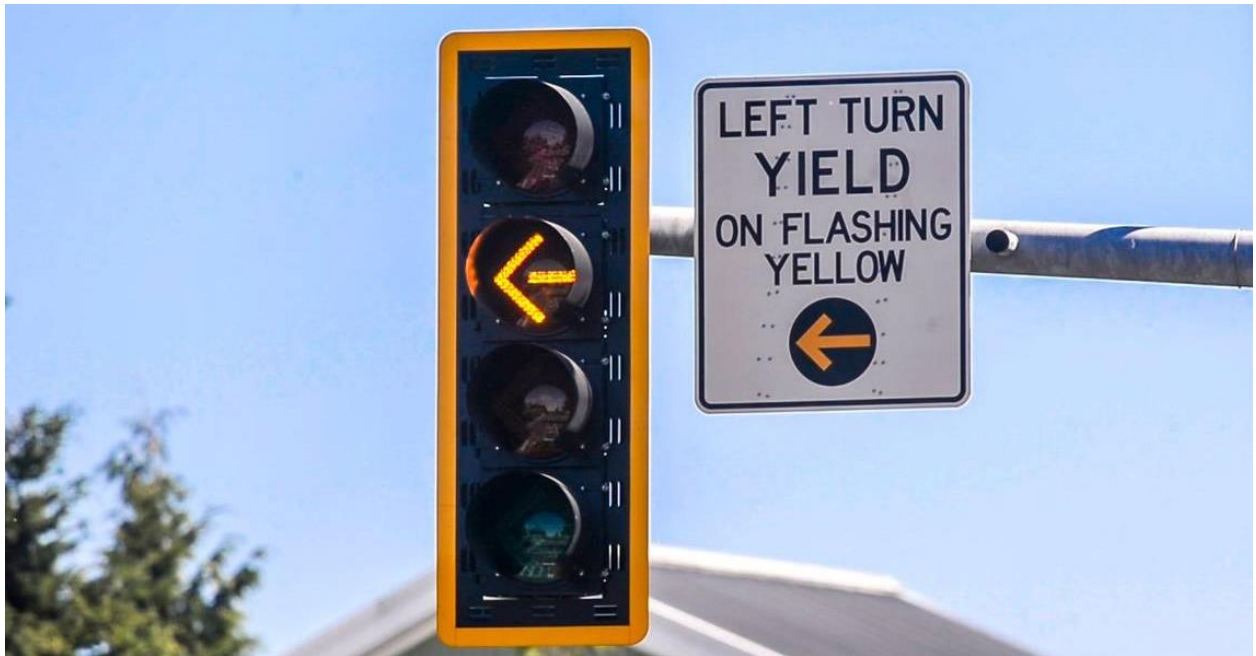
Figure 29: Flashing Yellow Left Turn Arrow with Yellow Retroreflective Backplate
