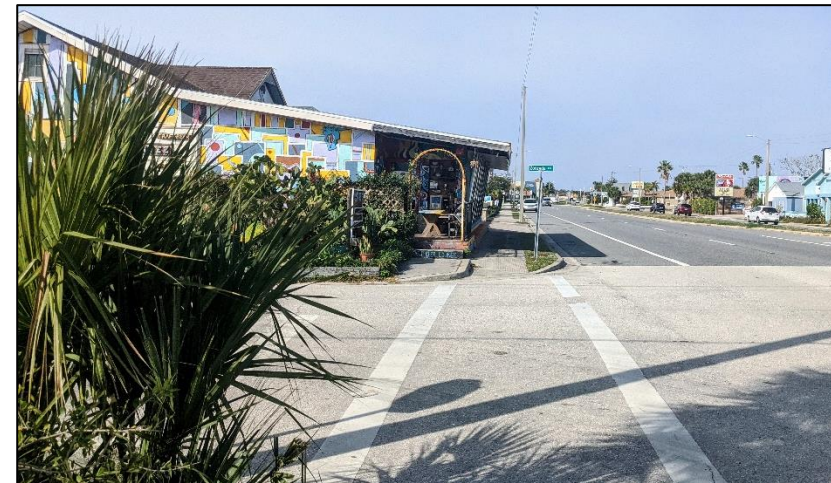
Example side street decorative crosswalk location on Zorayda Avenue adjacent to Sarbez. Source: Project Team.
