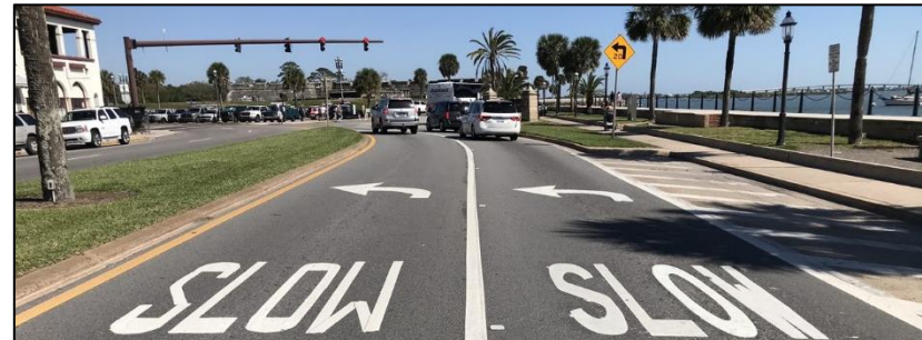
'Slow' pavement markings in downtown St. Augustine. Source: Project Team.
