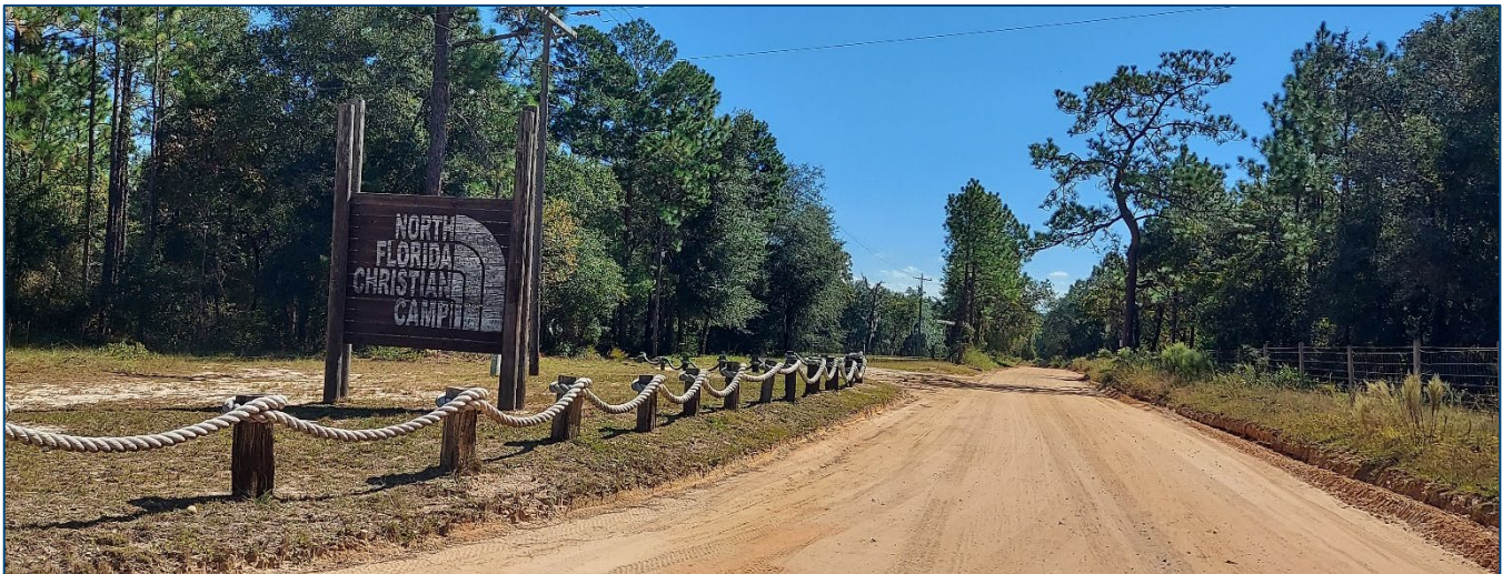
Christian Camp Rd in Keystone Heights is a prescriptive dirt road.
