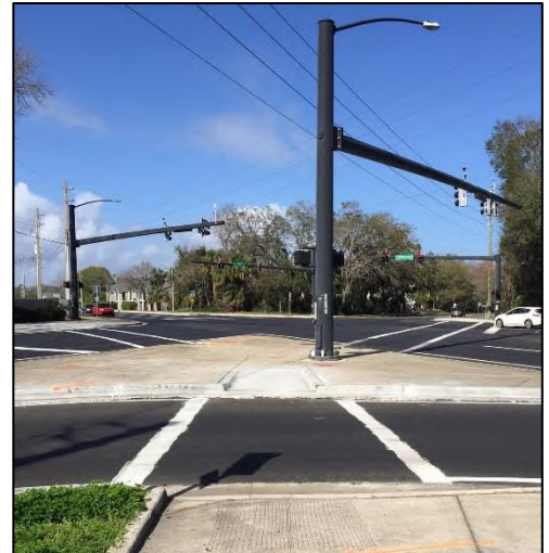
'Good' curb ramp at SR A1A/Wonderwood. Source: Project Team, February 2018.
