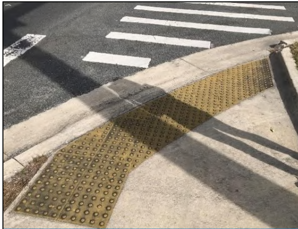
'Good' curb ramp at SR A1A/Mayport Road. Source: Project Team, February 2018.
