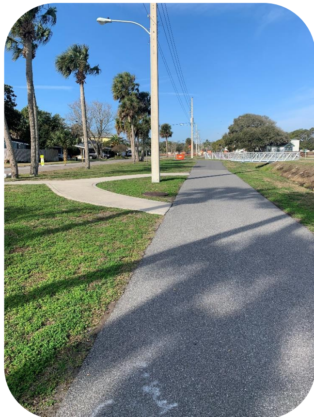
Existing trail along Florida Boulevard. Source: Project Team.
