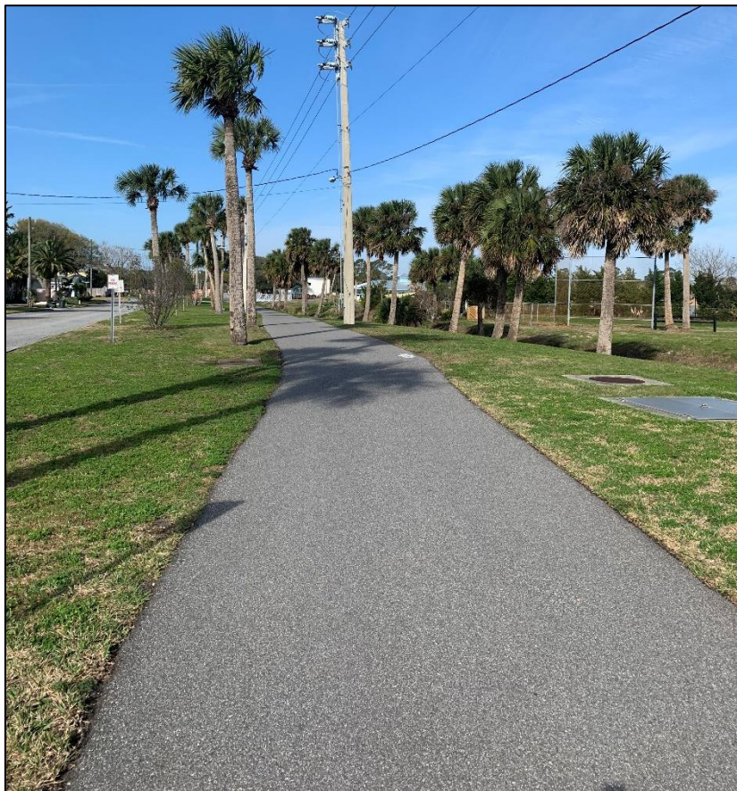
Existing shared-use path along Florida Boulevard. Source: Project Team.
