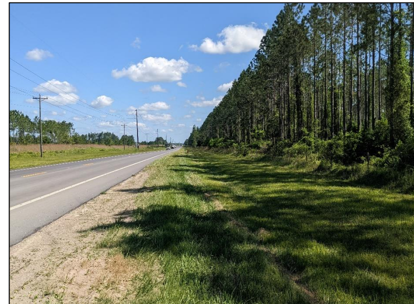
SR 21 in Segment 2. Source: Project Team.
