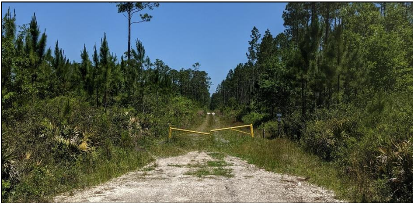
Existing service road (closed to public). Source: Project Team.
