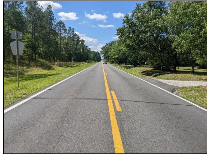
Long Bay Road near Old Jennings Road. Source: Project Team.
