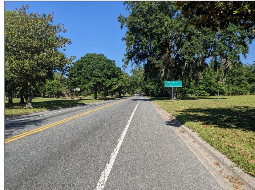
SR 16 west of CR 218. Source: Project Team.
