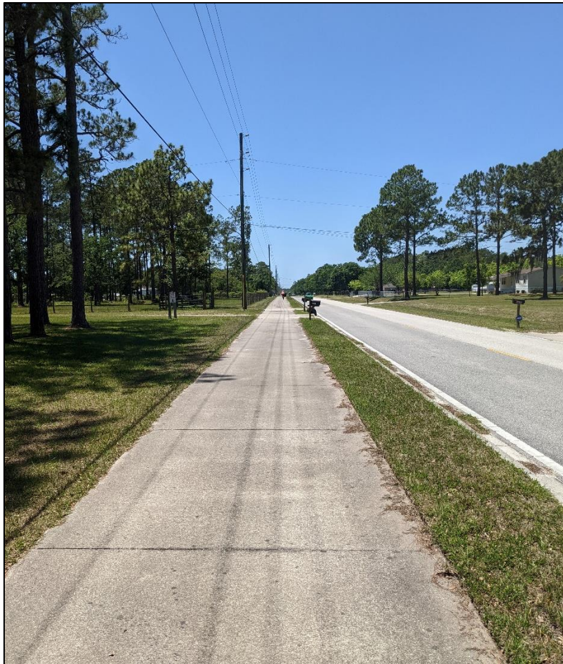
Existing sidewalk on Trail Ridge Parkway Source: Project Team.
