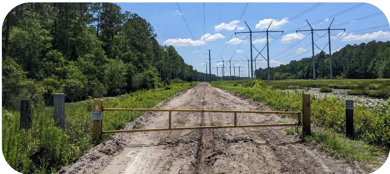
Utility corridor in Clay County. Source: Project Team.
