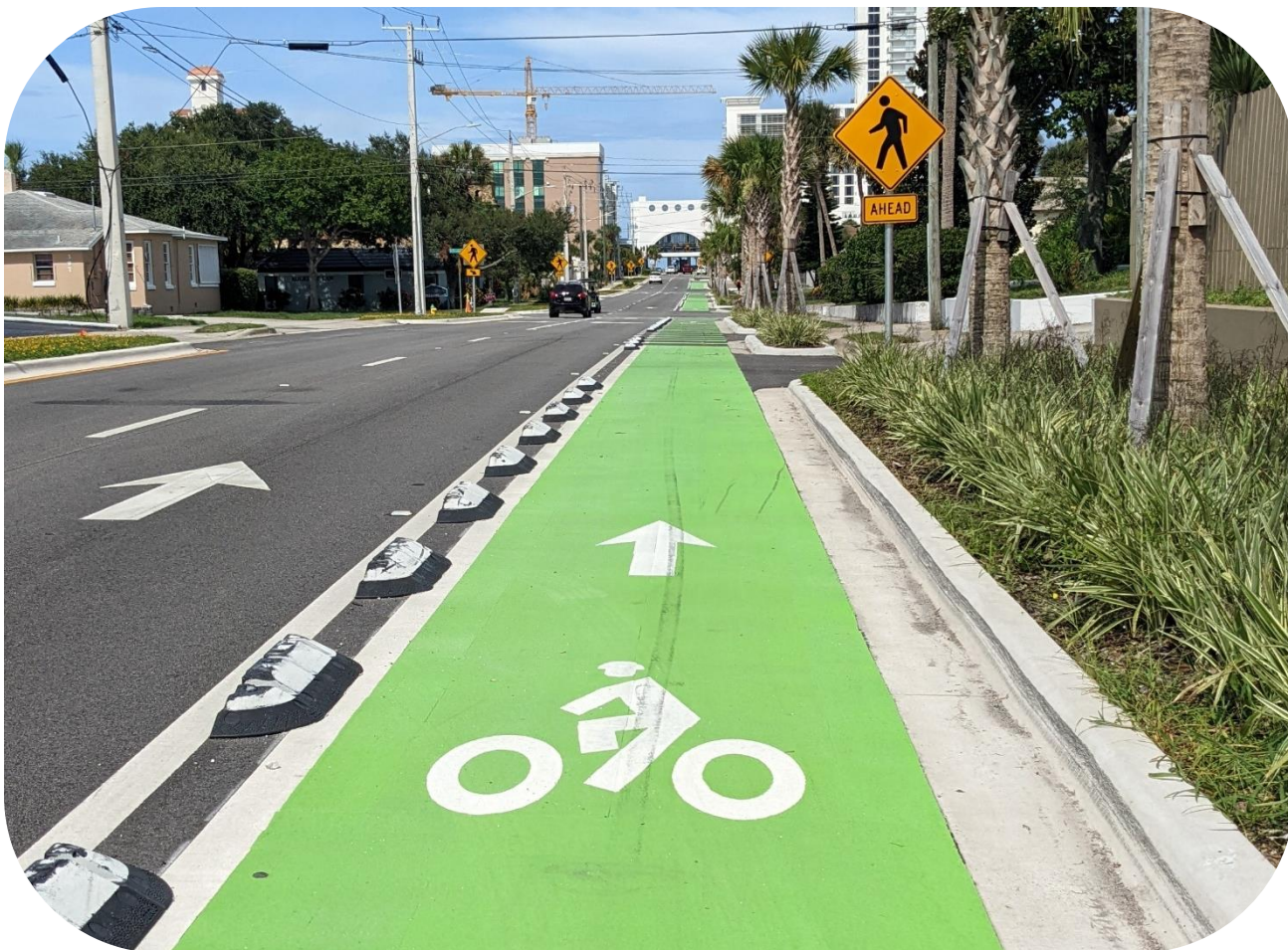
Protected bike lane in Daytona. Source: Project Team.
