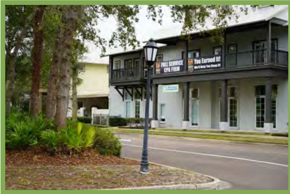
Pedestrian lighting along the east crosswalk (looking toward the southeast corner)
