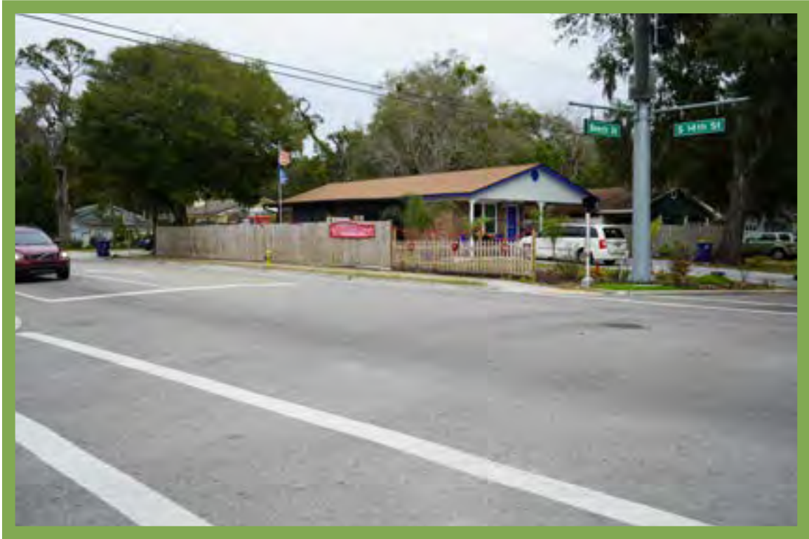
Looking toward the northeast corner
