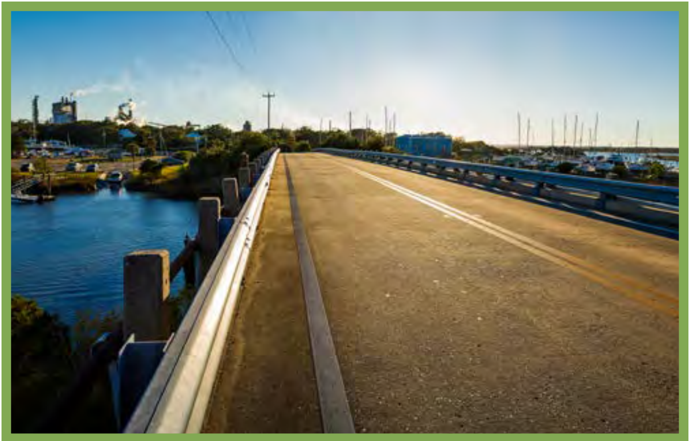
On the North 14th Street bridge (looking north)
