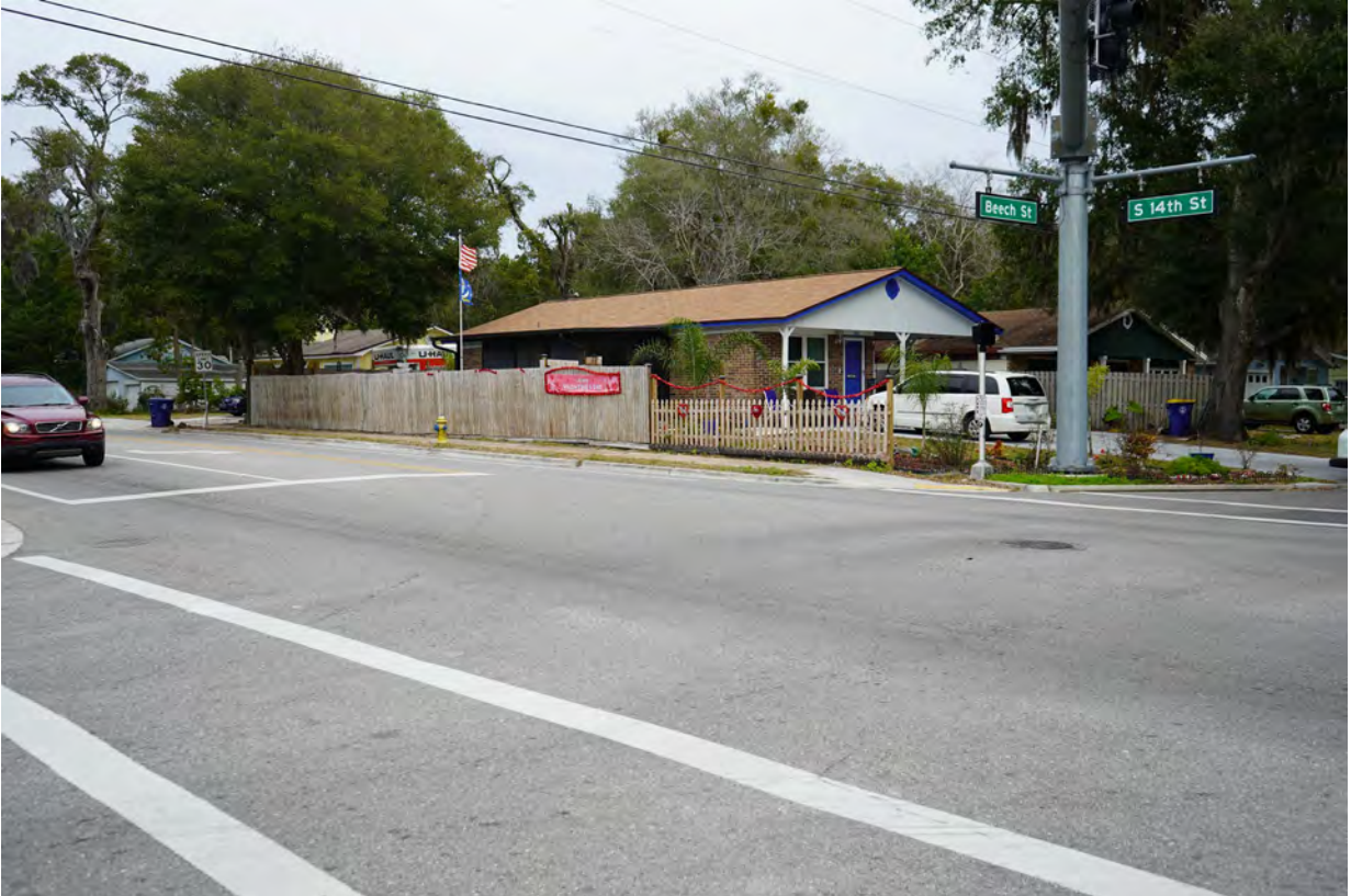
Photo: North side crosswalk is missing at the S. 14 th Street and Beech Street intersection
