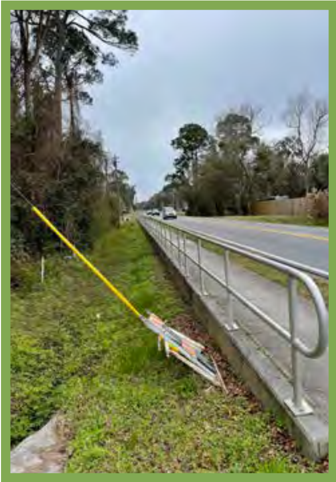
◀ Sidewalk along east side of 14th Street (southbound)
