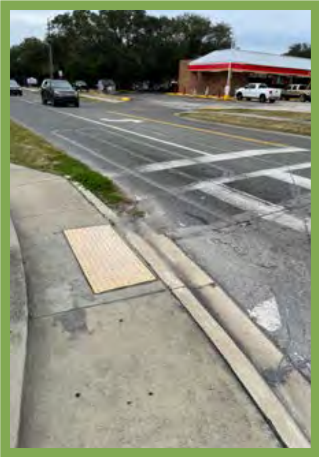
◀ Sidewalk ramp on the southwest corner
