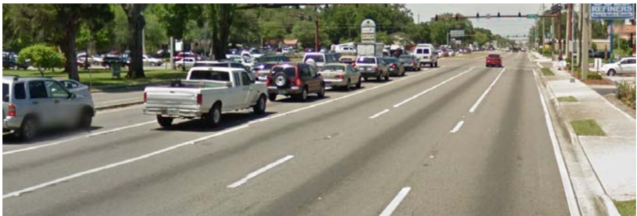
US-17/Park Avenue northbound, south of SR 224/Kingsley Avenue
