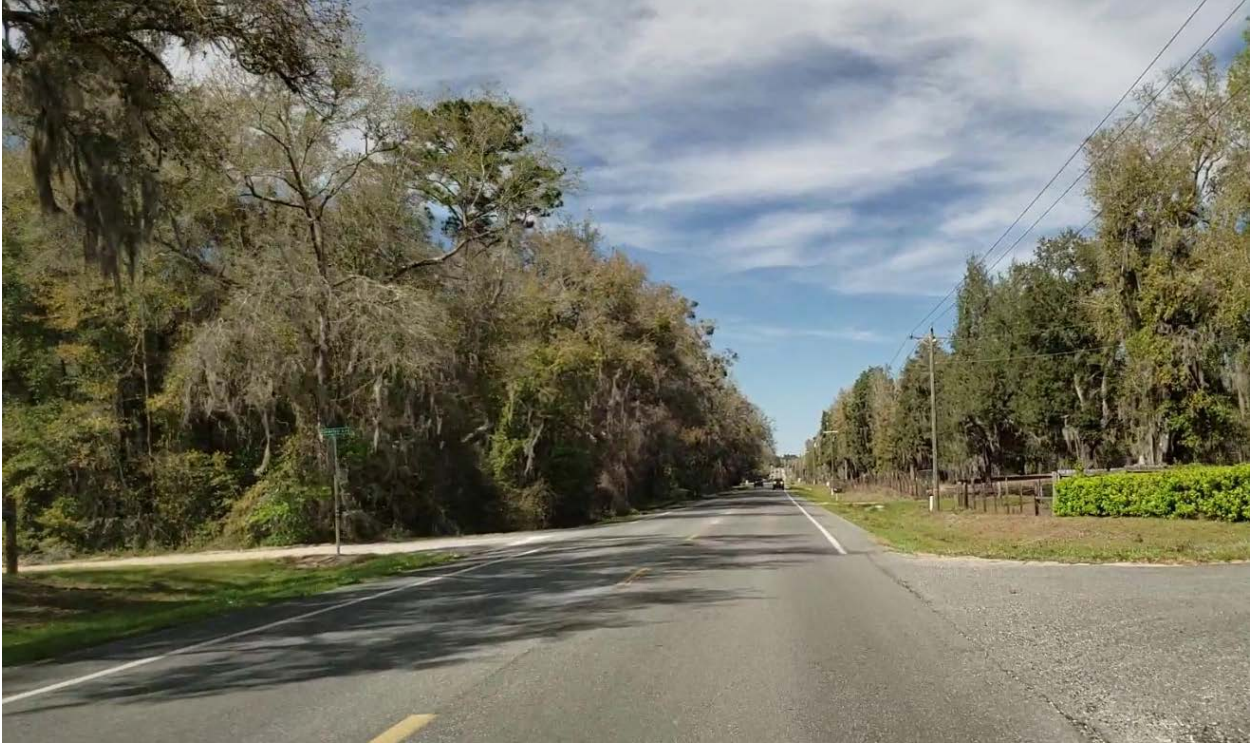
Figure 21. CR 315C Showing Oxidation and Shoulder Edge Wear
