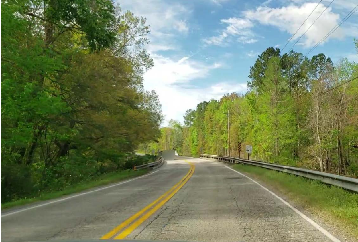
Figure 18. CR 220 near Little Black Creek Bridge
