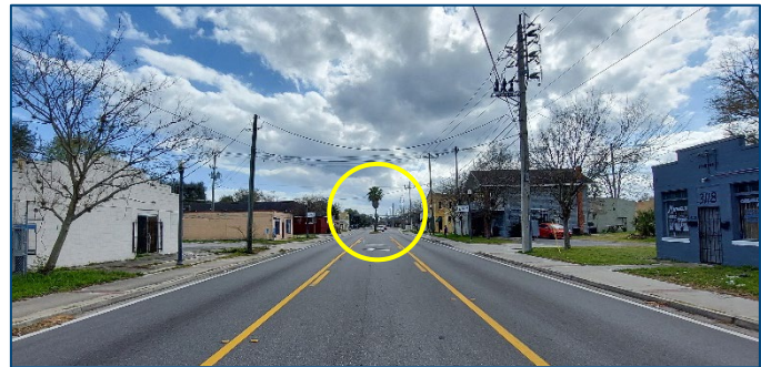
A cycle track on the northbound side of Myrtle Avenue is envisioned in this segment. The landscape island (circled in yellow) will be removed in the lane reallocation.
