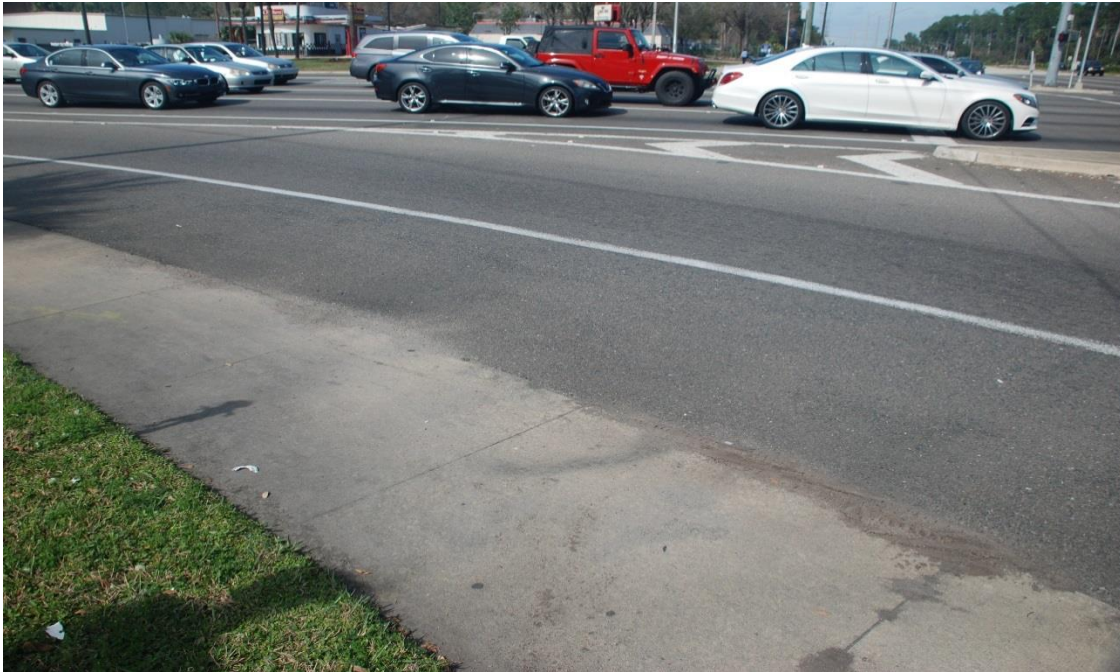
Sidewalk next to shoulder at Beach Boulevard and St. Johns Bluff Road (Also, as shown, a narrow sidewalk width of approximately four feet)
