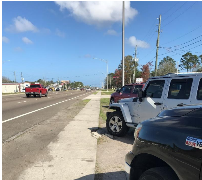
Beach Boulevard, between Southside Boulevard and St. Johns Bluff Road
