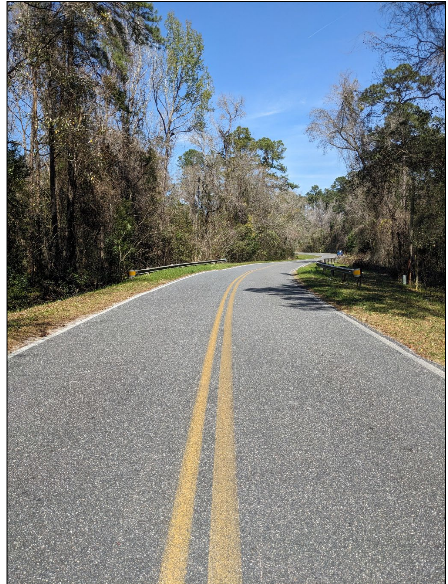
Typical view of Pine Street. Source: Project Team
