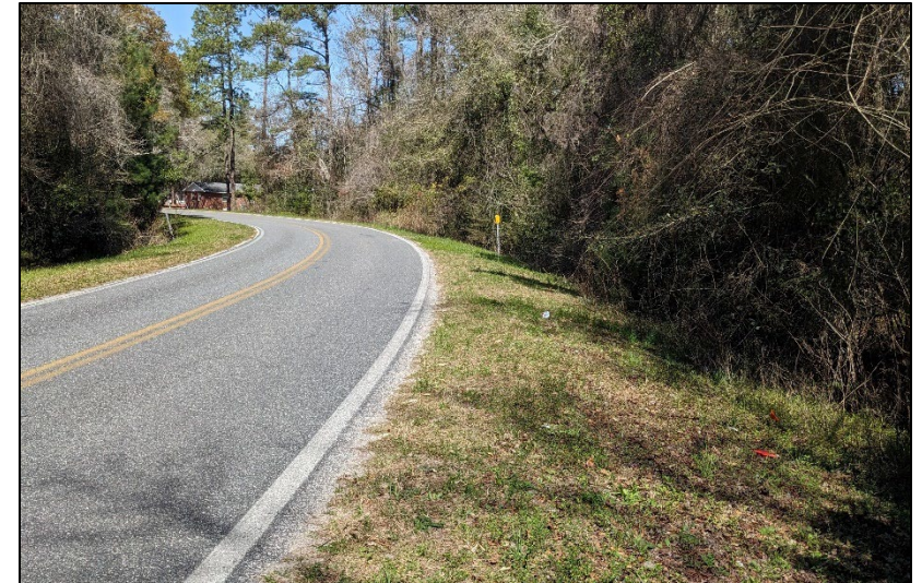
Example of a steep shoulder grade along Pine Street. Source: Project Team.
