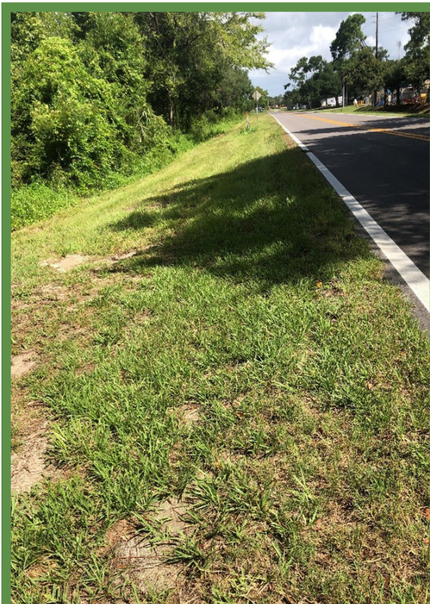
Old Dixie Highway (US 1 and Old Moultrie Road), Example of Potential Severe Slope Concerns (Gap ID 203)
