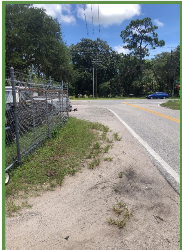
Hastings Road (Old Moultrie Road and SR 207) Example of Potential Right-of-way Concerns (Gap ID 204)
