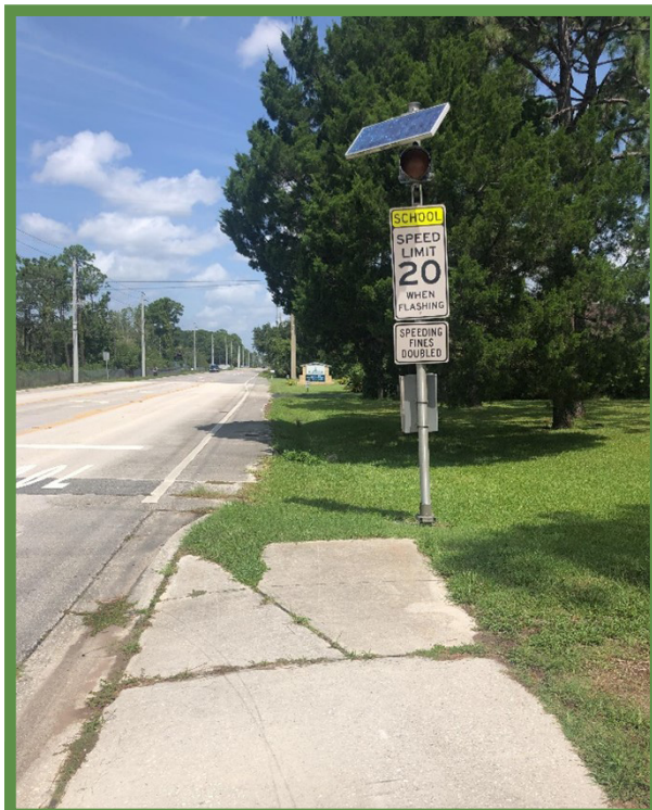
Sidewalk Gap on Lewis Speedway near Sebastian Middle School (Gap ID 155)
