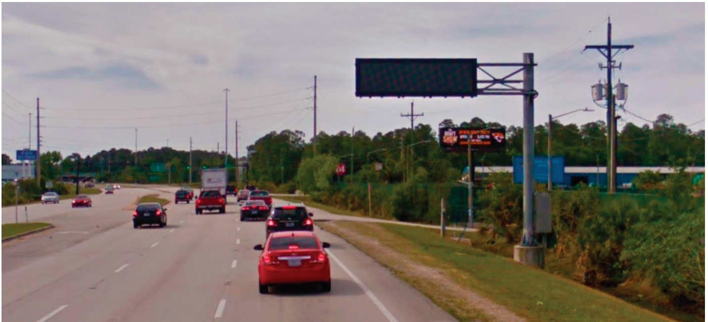
Example of Typical DMS Installation
