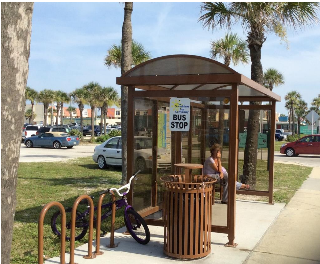
St. Johns County Pier Bus Stop, St. Augustine Beach
