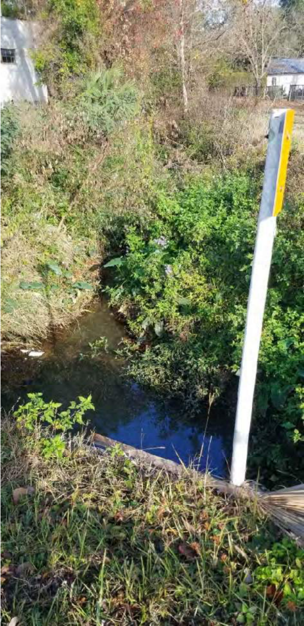
This is a photo of the FDOT drainage structure (culvert inflow) conveying pond outflows and drainage from beyond Drew Street. Here is a view of the channel downstream of the 10-foot by 5-foot culvert.
