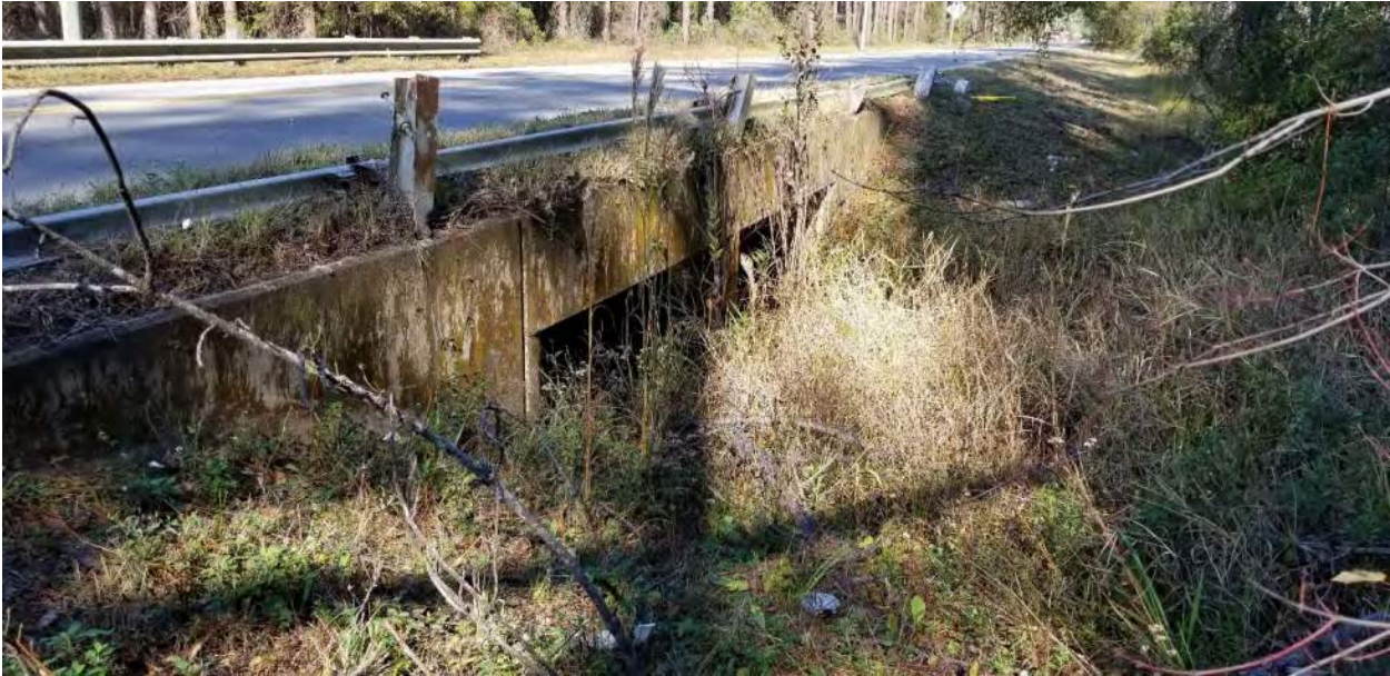
Existing culvert under Yellow Water Road (upstream).
