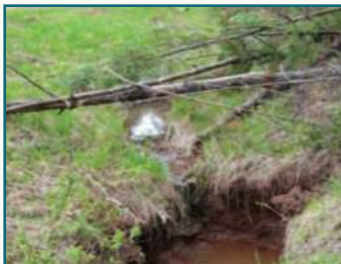
Ditch obstruction/ blockage
