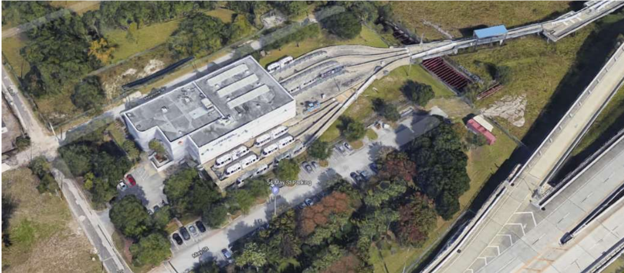
Figure 5: The JTA's Skyway Operations and Maintenance Center
